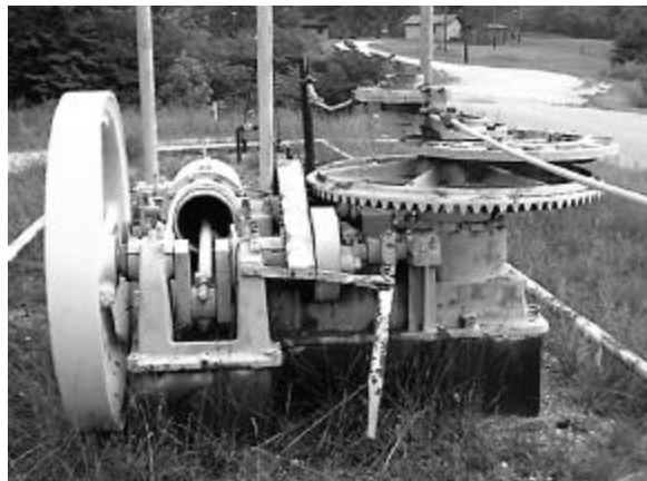
A one-cylinder natural gas engine provided power to produce multiple wells via attached rod lines.
